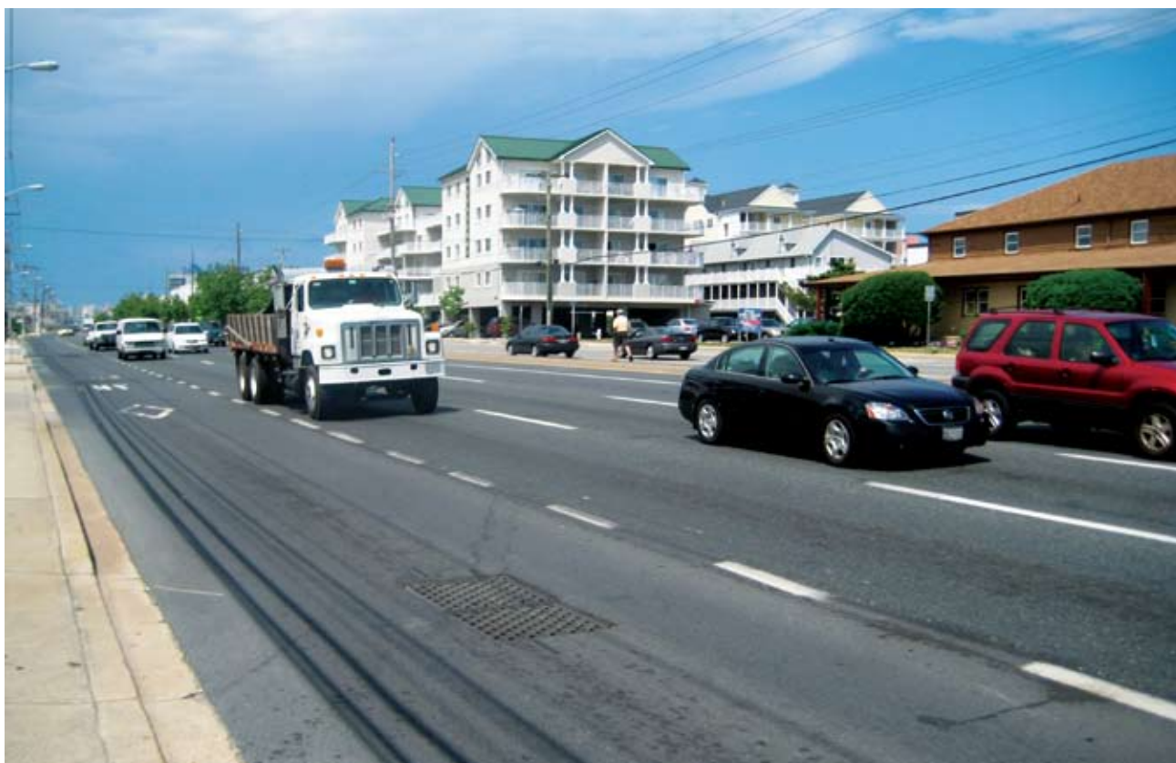
Ocean City, Md., sees traffic increase tenfold during the prime summer vacation season. HDPE pipe installed in 1987 has improved drainage for the past 24 years.
