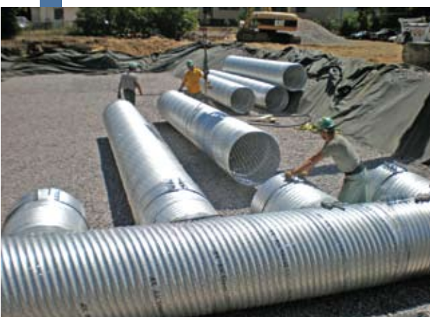
Subsurface installation in Wisconsin.
