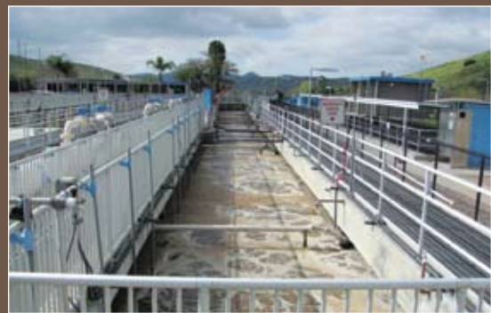
The anoxic zone of the biological nutrient removal treatment process uses microorganisms to rid the water of pollutants.
