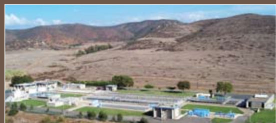
The plant provides recycled water to the Santee Lakes for recreation and to local parks, schools and greenbelts for irrigation.
