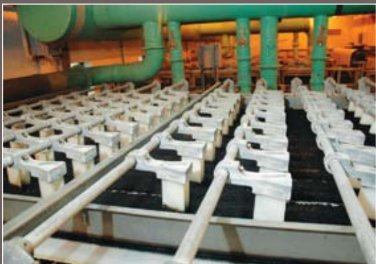
The facility plans to become self-powering and eventually contribute surplus energy to the grid.
