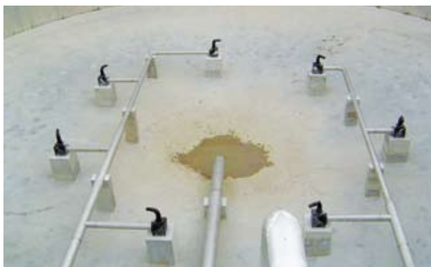
The JetMix system's nozzles can be rotated 360 degrees, allowing operators to effectively mix material and keep it in suspension, even in hard-to-mix tanks.
