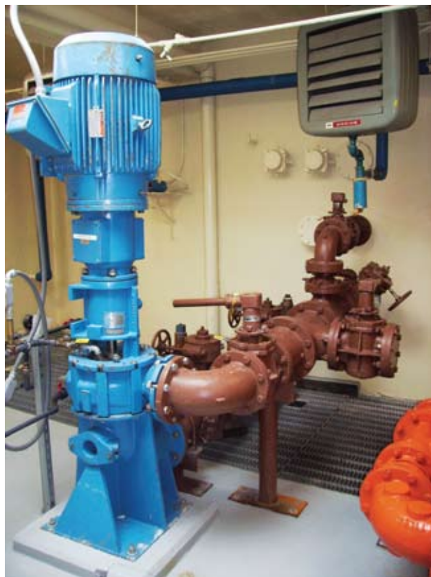
A vertical chopper pump helps break down rags and other solids into smaller particles, reducing clogs and making digestion easier.
