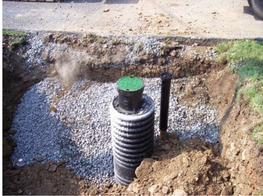
The sewer main lining installation.
