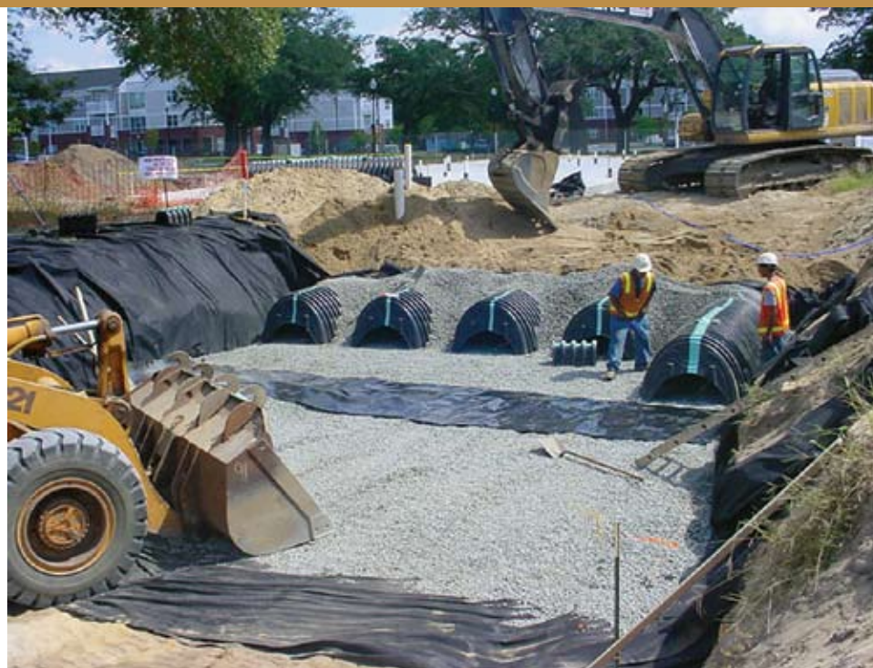
Sites for the system's five beds were planned carefully to avoid disturbing building foundations and old oak trees.
