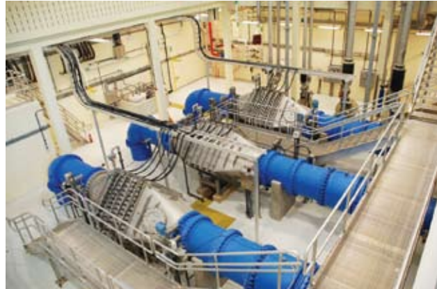
Left: The ozone system consists of two ozone generators. The units alternate in operation with one duty unit online while the other remains on standby. Right: The use of UV technology for drinking water disinfection represents a trend away from reliance on chemical disinfection and will enable the new plant to comply with more stringent federal disinfection byproduct rules.
