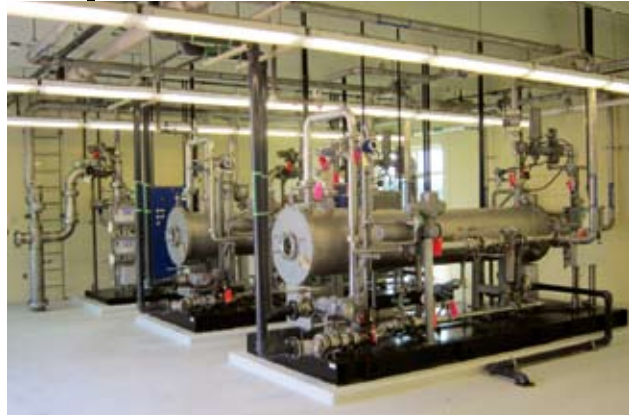
Left: The ozone system consists of two ozone generators. The units alternate in operation with one duty unit online while the other remains on standby. Right: The use of UV technology for drinking water disinfection represents a trend away from reliance on chemical disinfection and will enable the new plant to comply with more stringent federal disinfection byproduct rules.
