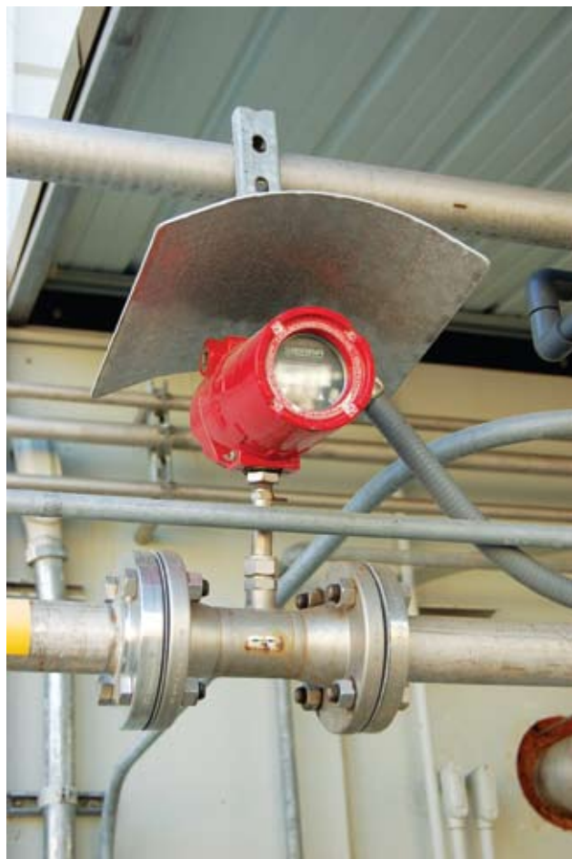
Using its new thermal technology, the WWTF can measure true mass flow with 40:1 rangeability.
