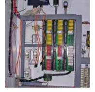
The new control system is 100 times faster and offers improved PID handling capabilities and higher-density I/O.
