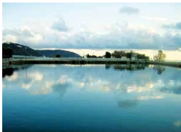
Drinking water is stored in reservoirs, usually located on high ground.
