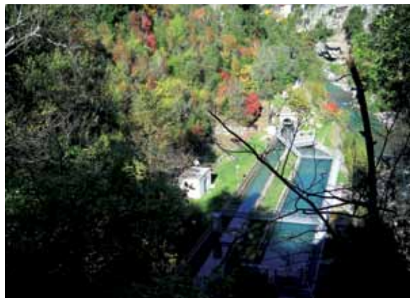
The Super-Rimiez Plant is at the forefront of potable water production sites in Europe, with nine production centers and a capacity of 460,000 cu meters per day.
