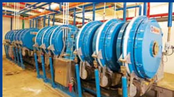
Two new rotary sludge presses were installed.
