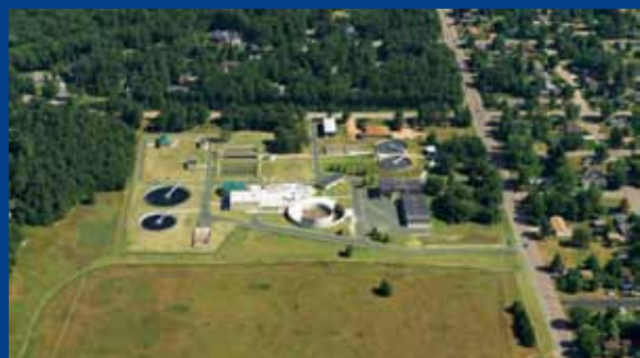
Wisconsin Rapids WWTP conducted $23.8 million in facility upgrades to meet the evolving wastewater needs of industrial customers.
