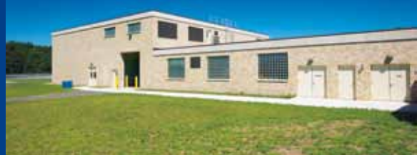
The south side of the sludge handling building, home to a biogas engine generator.
