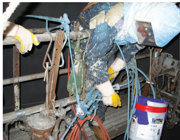
Workers applying primer with optically active pigment
