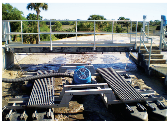
The aerator and mixers provide dual functionality, which can save on operating and energy costs.
