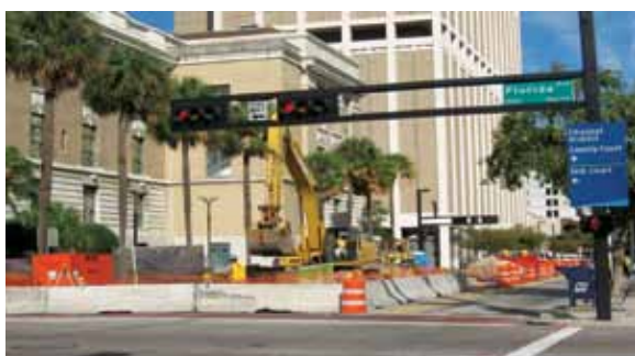
Numerous cities throughout the U.S. are using design-build and design-build-operate methods on water and wastewater improvement projects.
