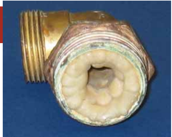
Limescale deposits can form wherever water is heated.
