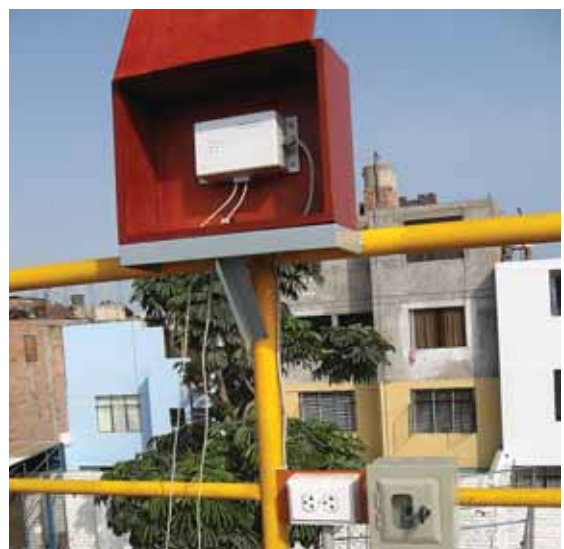
Electronic devices cause existing scale deposits to soften and subsequently be removed from the system.
