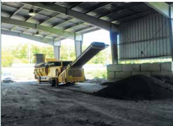
Stockpiled sludge is aged for three years and will be turned over several times during that period when stockpiles are rearranged.
