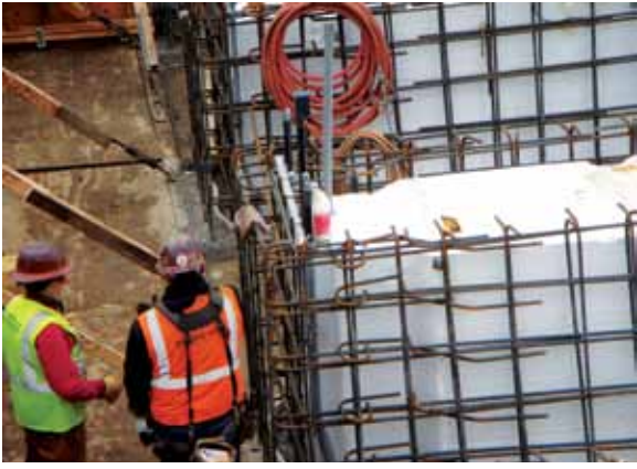
EPS geofoam is approximately 98% air and 100 times lighter than soil.
