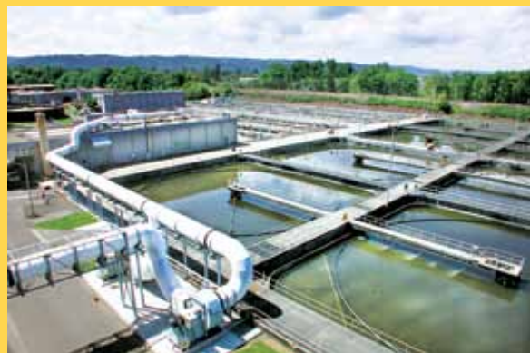
Wet weather clarifiers
