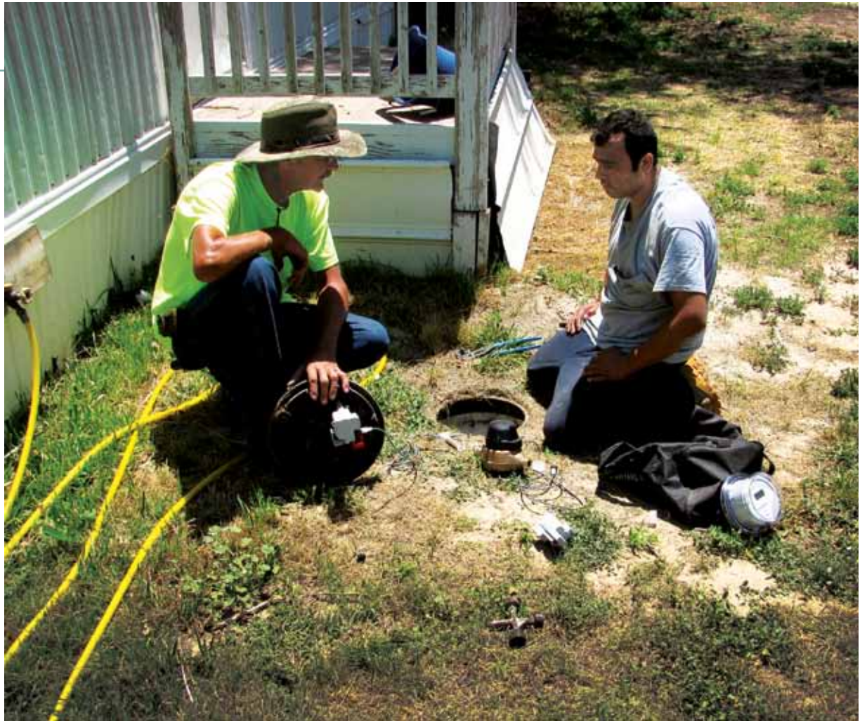
A crew installs a residential water meter as part of a new AMR system.
