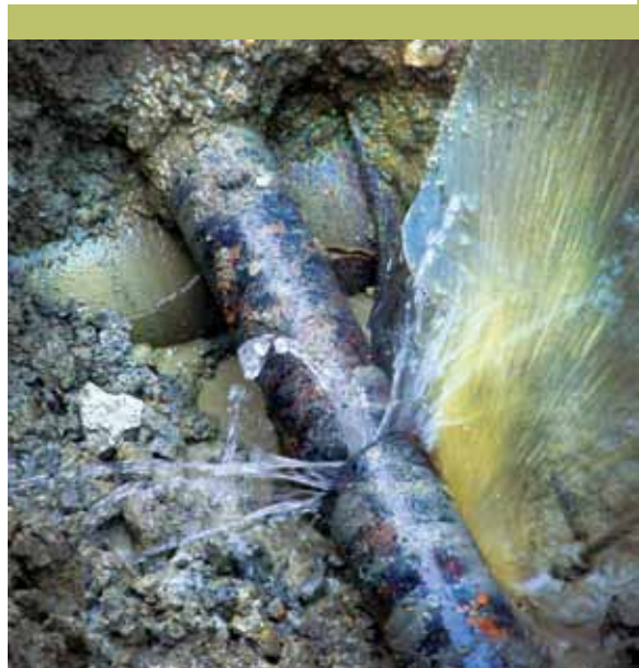
Specialized equipment is capable of “listening” to leaky pipe.
