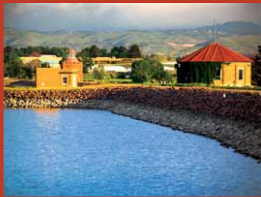
The Marston WTP was built in 1924 and sits at the edge of a reservoir.
