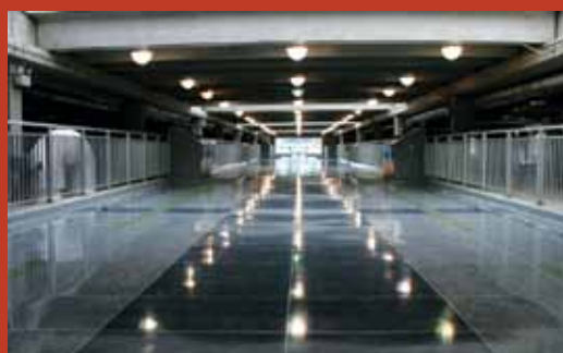
Future Marston WTP upgrades include replacing and upgrading the flocculators and solids removal equipment.
