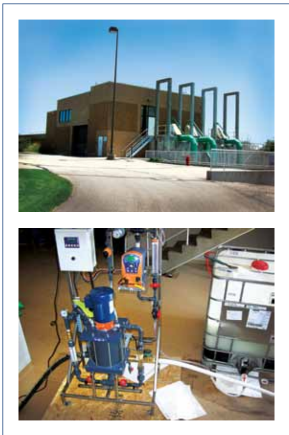
Based on a three-week performance trial, Greeley, Colo., elected to install a polymer feed system resulting in a drier cake production and reduced polymer consumption.
