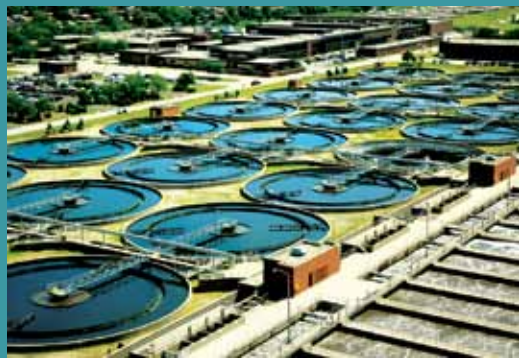
The Stickney WRP is the largest wastewater treatment facility in the world.
