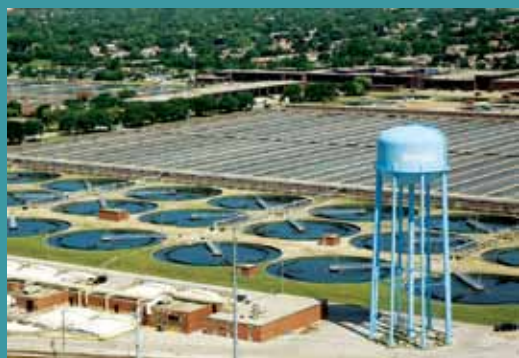
Upgrades will reduce solids carryover in recycle streams and thicken solids more efficiently.
