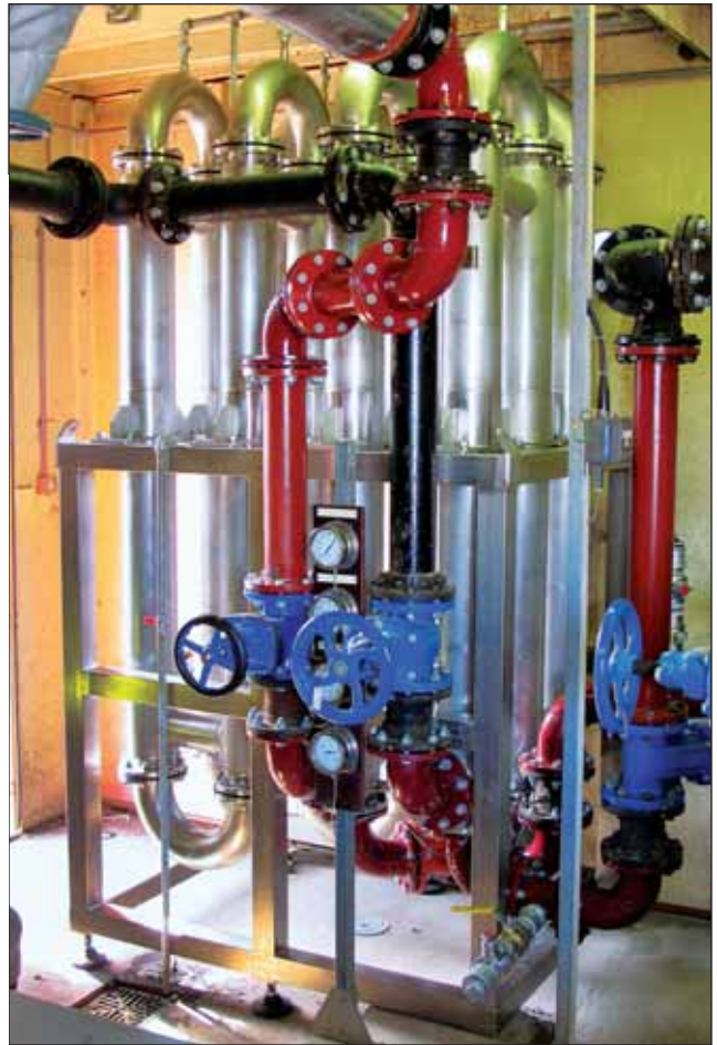
Corrugated double tube heat exchangers have a successful track record in handling waste streams.
