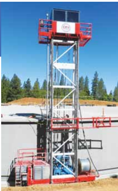
The strandwrapping/shotcrete machine ensures long-life, liquid-tight structures.
