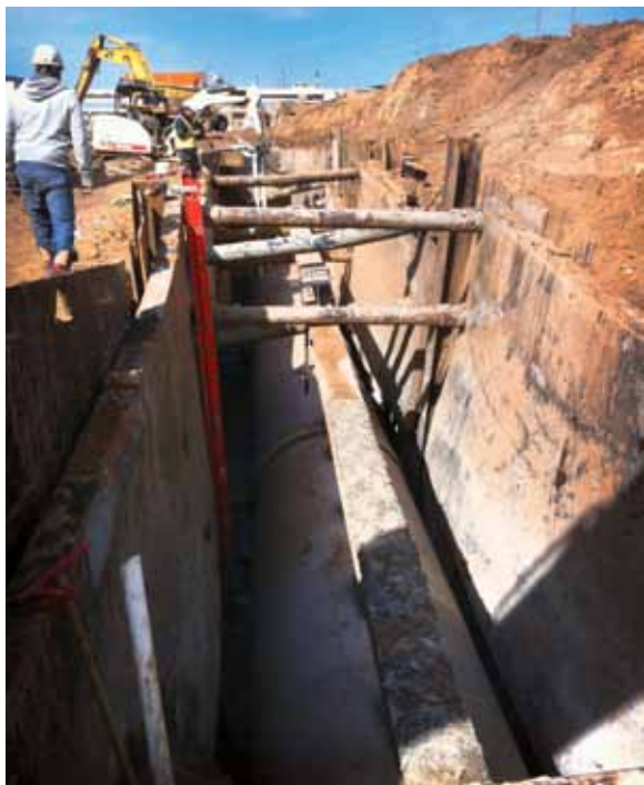
The pipe was installed under the Oklahoma River.
