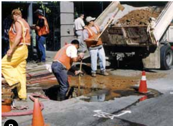
B Street excavation
