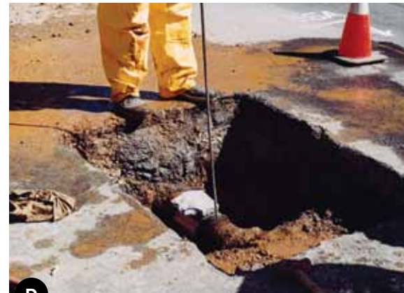
D Conducting a final check
