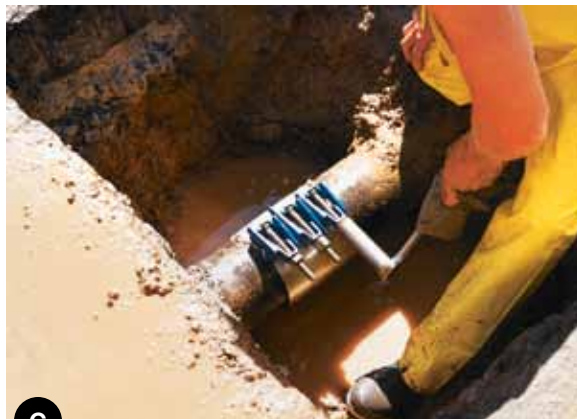
C Utilizing a repair clamp
