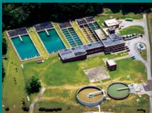
The plant serves 37,000 metered customers and provides an average of 15 mgd.
