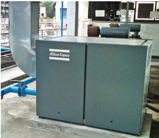
After experiencing reliability problems with its lobe blowers, Sandoz decided to shift to the new technology of screw blowers.
