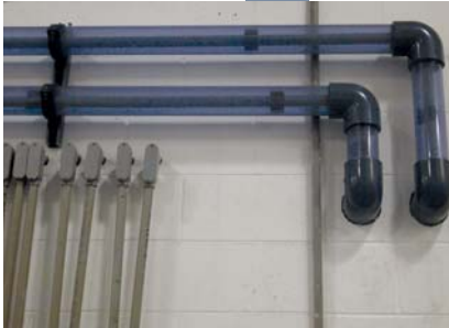
The clear outer containment pipe allows visual leak detection.
