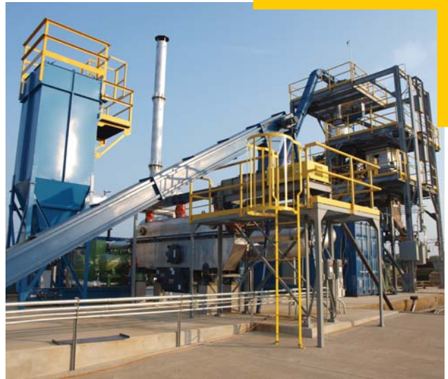
Overview shot looking from the dryer back toward the gasifier
