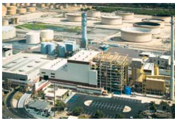
Plant view facing north
