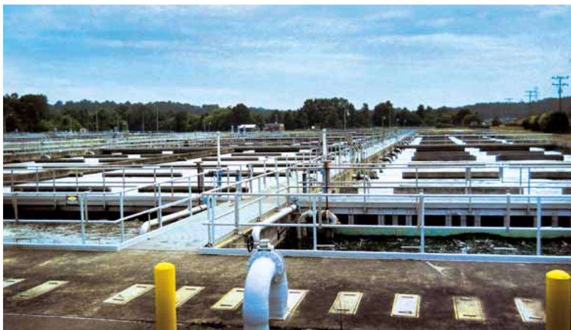
Upon completion, the new aeration system at CCUC's Archie Elledge WWTP is expected to yield energy savings of approximately $117,000 per year, which will provide a simple payback of six years.
