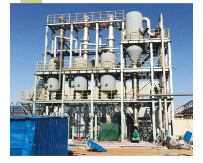
vast amounts of water needed for plant process and discharge and strict regulation of wastewater discharge, the biggest challenge for the Mengda project is to achieve its goal of zero liquid discharge (ZLD), meaning no contaminants from the manufacturing process will get into the groundwater system.
