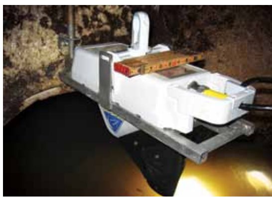
Crews installed more than 155 meters in 45 days to get the program up and running.
