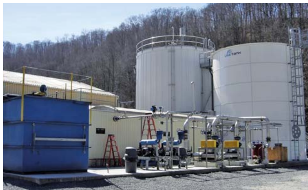
Left: Membrane tank Below: The AnMBR and MBR system
