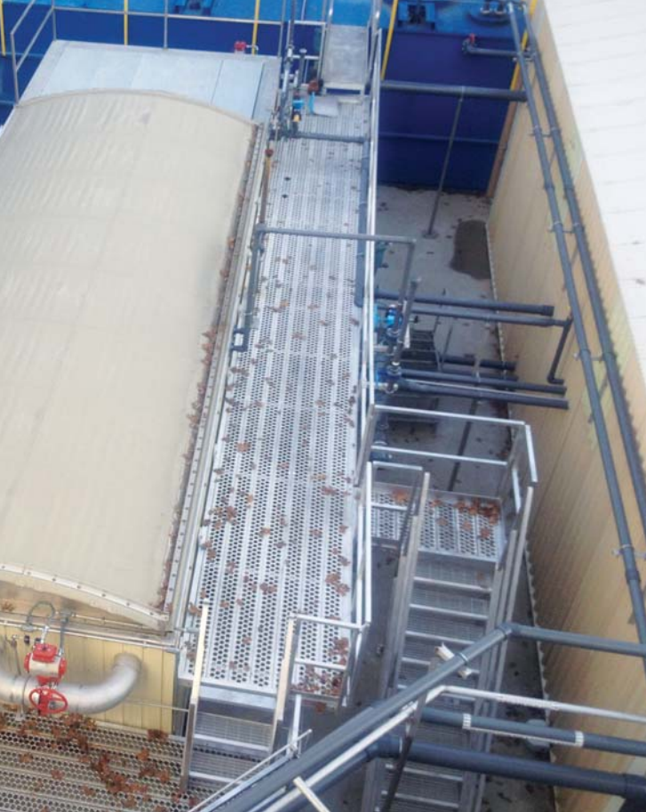
Left: Membrane tank Below: The AnMBR and MBR system
