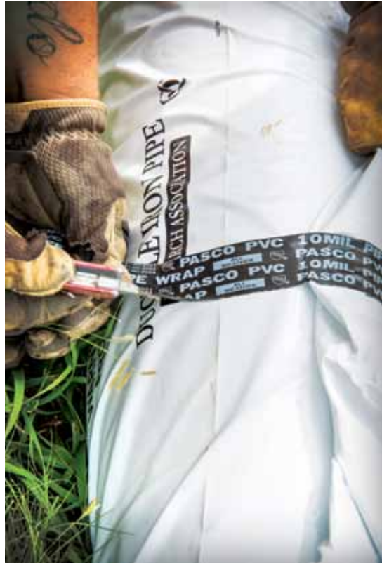
The encasement is infused with an anti-microbial and a corrosion inhibitor.
