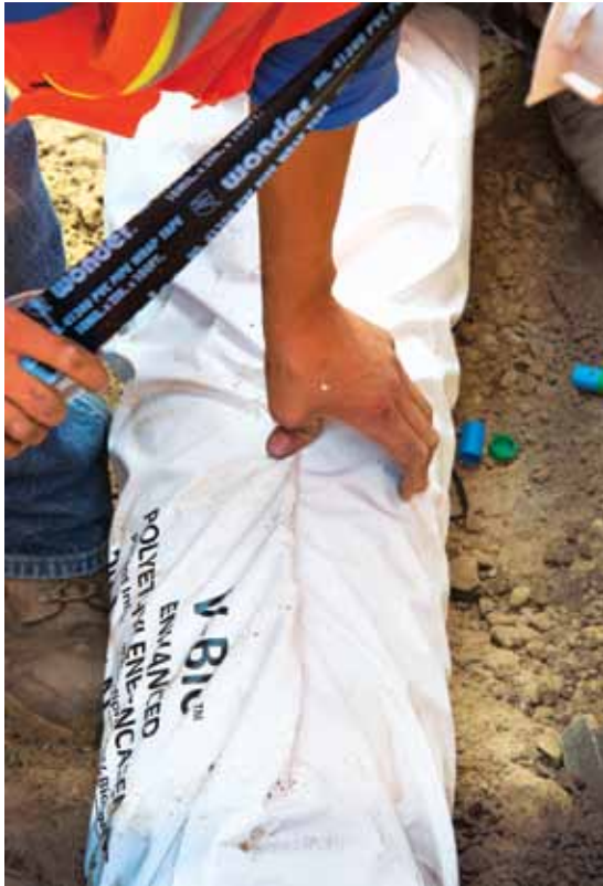
The polyethylene encasement is used to protect iron pipeline from aggressive soils.
