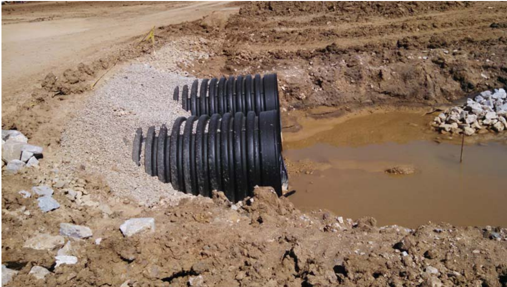
More than 2 miles of large-diameter corrugated HDPE pipe were installed.
