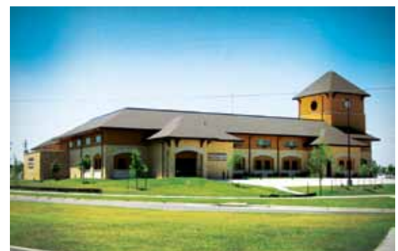
The Hutchinson plant was built in 2008 and treats 10 million gal per day, providing water to 41,000 residents and businesses.
