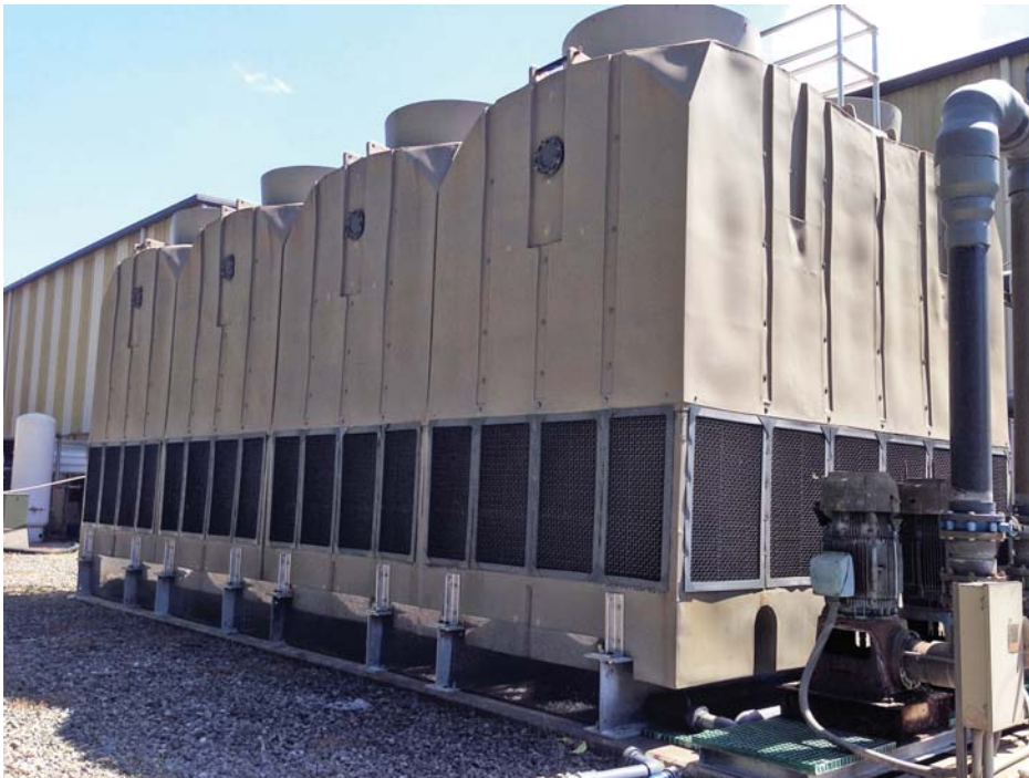
HDPE-engineered plastic cooling towers address corrosion problems that plague metal towers due to soft water, aggressive water treatment and ambient factors like caustic industrial gases.
