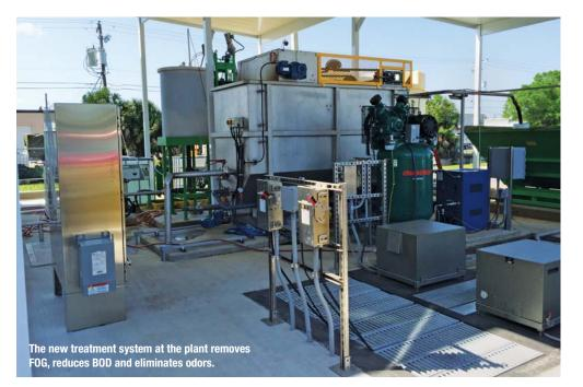
treatment system that included an equalization tank, continuous removal of free-floating fats, chemical reaction tanks, a dissolved air flotation (DAF) system and sludge dewatering. The entire system was designed and fabricated in-house, as was the handling of the wastewater system permitting process for the client.
