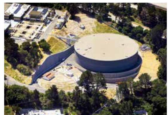
The 11-million-gal treated water reservoir was built to withstand earthquakes along nearby faults.
