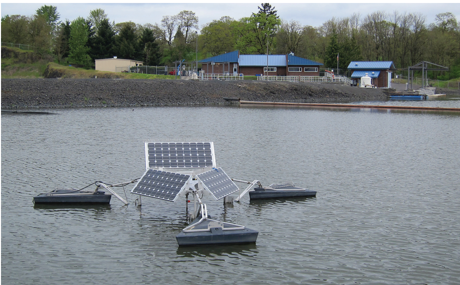
SolarBee solar-powered mixers help reduce aeration runtime and improve mixing.
