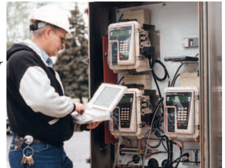
With solar power and radio communications, these 950AVs monitor three billing sites.
