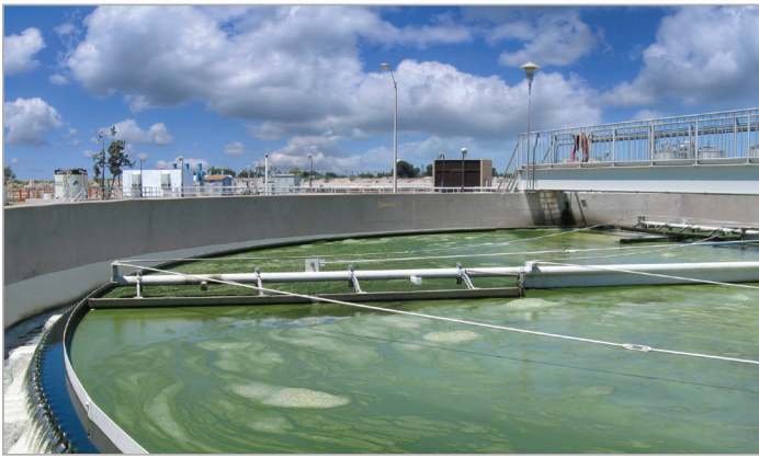
Algal Bloom Dissolved Air Flotation Treatment
