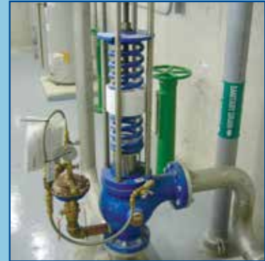
Region of York (Nobleton) installation Ontario, Canada
