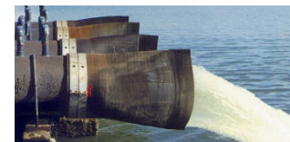
Figure 4 - An Elastomeric “Duckbill” Tideflex ® Check Valve Flowing
