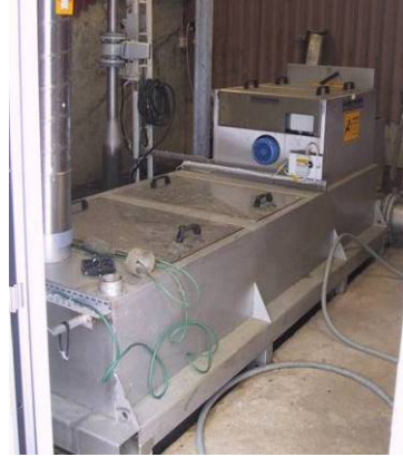
Figure 15 – Tank mounted Step screens
