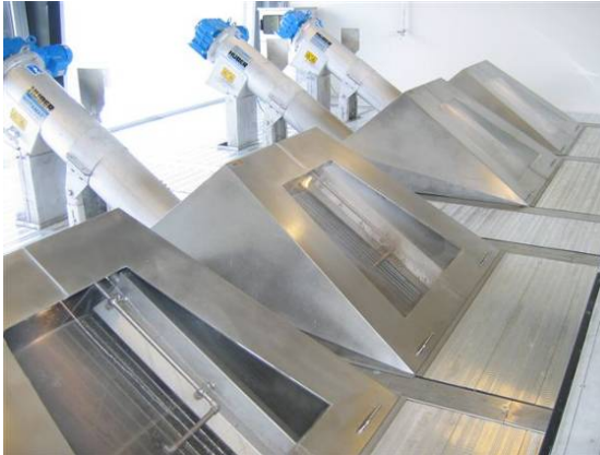
Figure 3- Ro2 installation in Denmark
