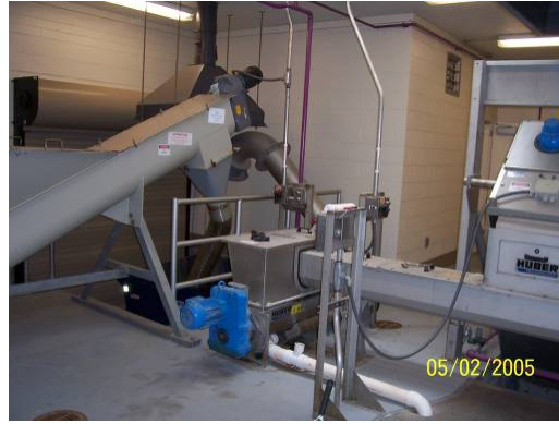
Figure 7- Step Screen at Gardner, KS
