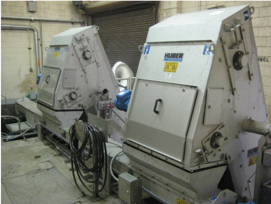
Escamax Perforated Plate “Double Pass” Screen
