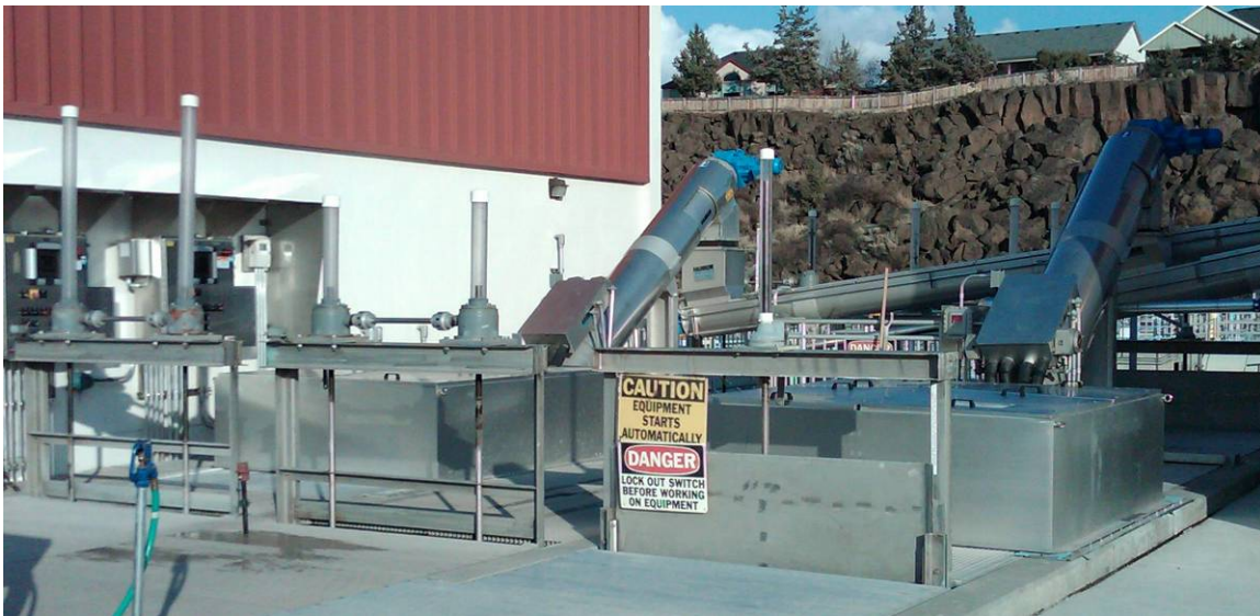
Rotamat® RPPS Center Feed Drum Screen
