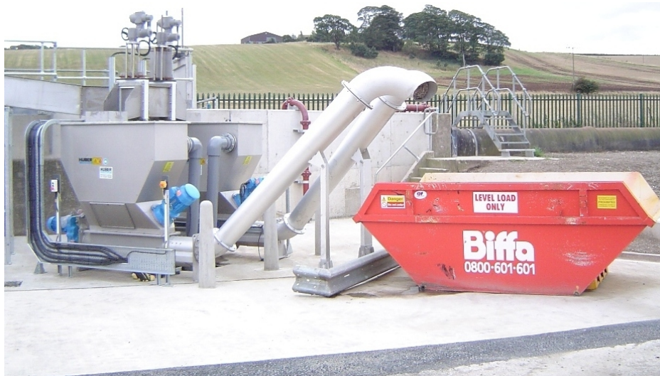
Figure 38 – Screenings washer/compactor with launder feed - Clayton West, UK
