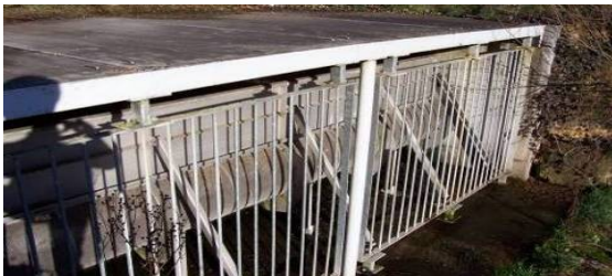
Figure 28 – Installation underneath a gutter
