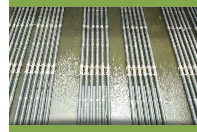
StreamLine provides full solids suspension both above and below the diffuser grid. Elevation of the diffuser is adjustable to match blower performance.
